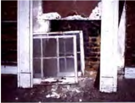
Loose or detached elements should be identified, tagged and stored, preferably on site. Photo: NPS files
