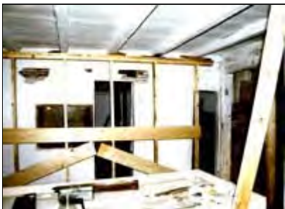
Interior bracing which will last the duration of the mothballing will protect weakened structural members. Photo: John Milner Architects.
